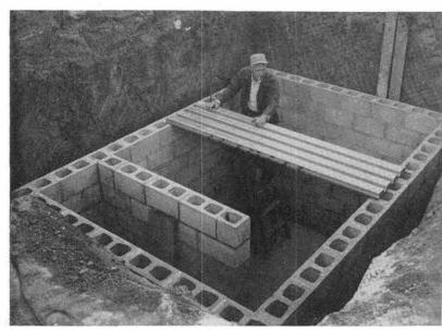
CHUCK PIGNOLET (8161-2) adjusts one of the steel ceiling supports on his fallout shelter before topping it off with six inches of reinforced concrete and two and one half feet of earth. The shelter is designed to meet Civil Defense specifications.
